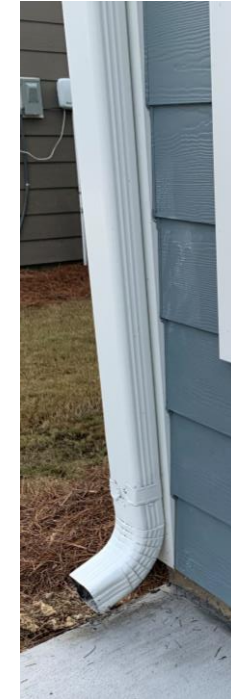
GUTTERS Included on front and rear of house.
