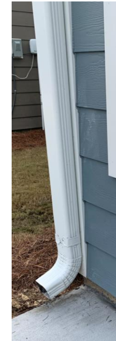
UPGRADES Gutters on front and rear of house.
