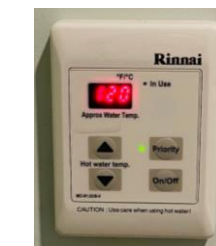
WATER HEATER Rianni Tankless Water Heater Exterior location temp control
