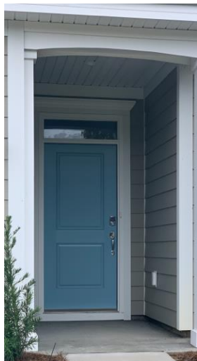
FRONT DOOR Included Front Door
