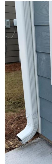
GUTTERS Included on front and rear of house.
